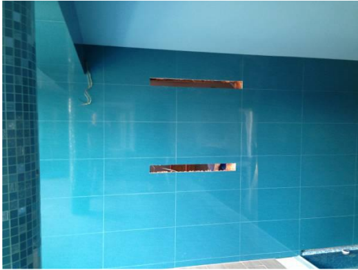
1. Cutting wall transitions
