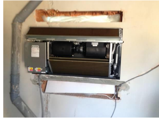
4. Installation of dehumidifier and connection of electric cable and condensate drain
