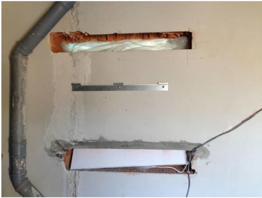
3. Wall console assembly
