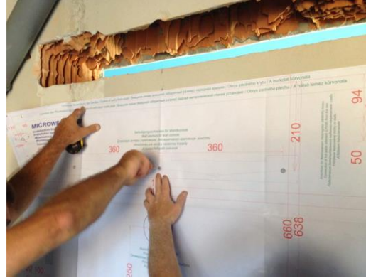
2. Console measuring using template
